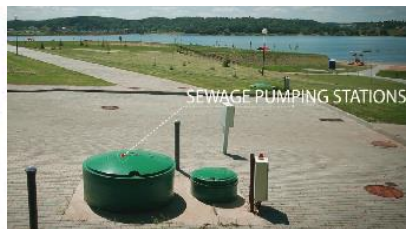
Water supply system, 3 sewage pumping stations with a capacity 24 m 3 /h
